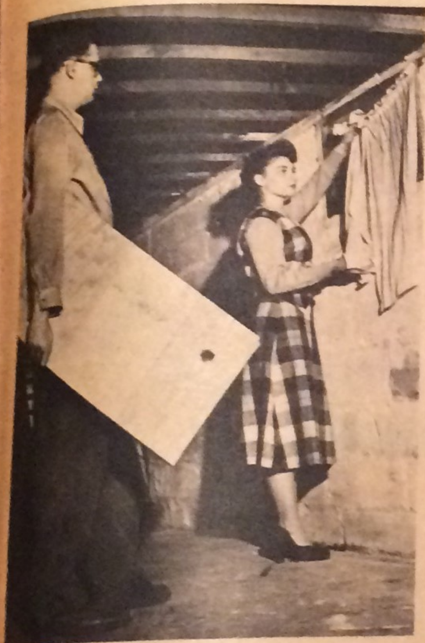
Curtains and all inflammable material should be removed from the shelter area and exposed wood covered with fire-retardant paint.
