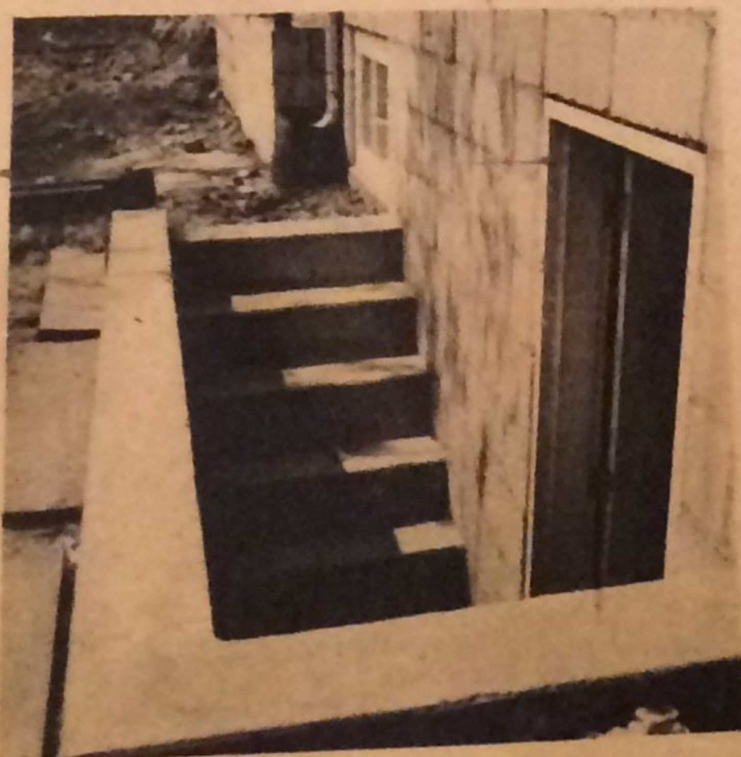
A completed basement exit project, with concrete block retaining wall capped by cement. Pre-cast concrete steps are available.
